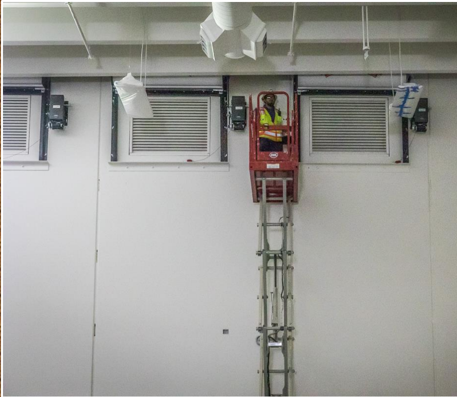
Hat channel being installed to receive acoustical panel
